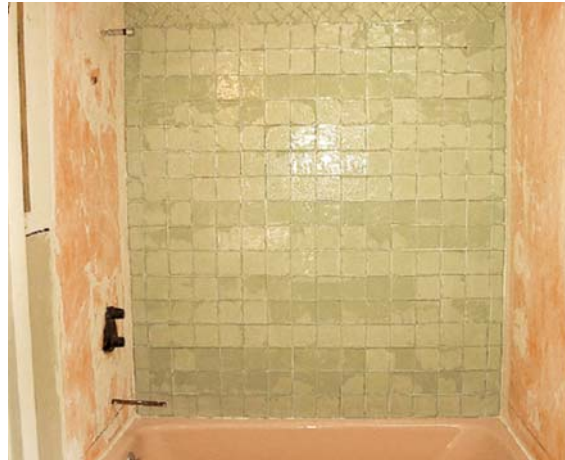
A mottled bond coat pattern may become visible through translucent or transparent glass tiles when they are installed over a waterproofing membrane.
